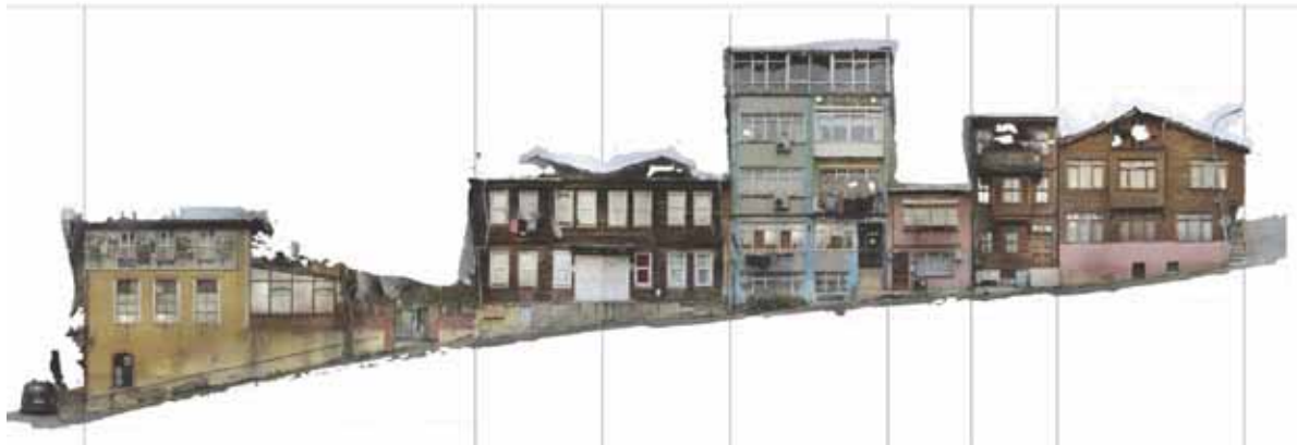
Fig.1. Buildings block number 456 facing Meydan Street
